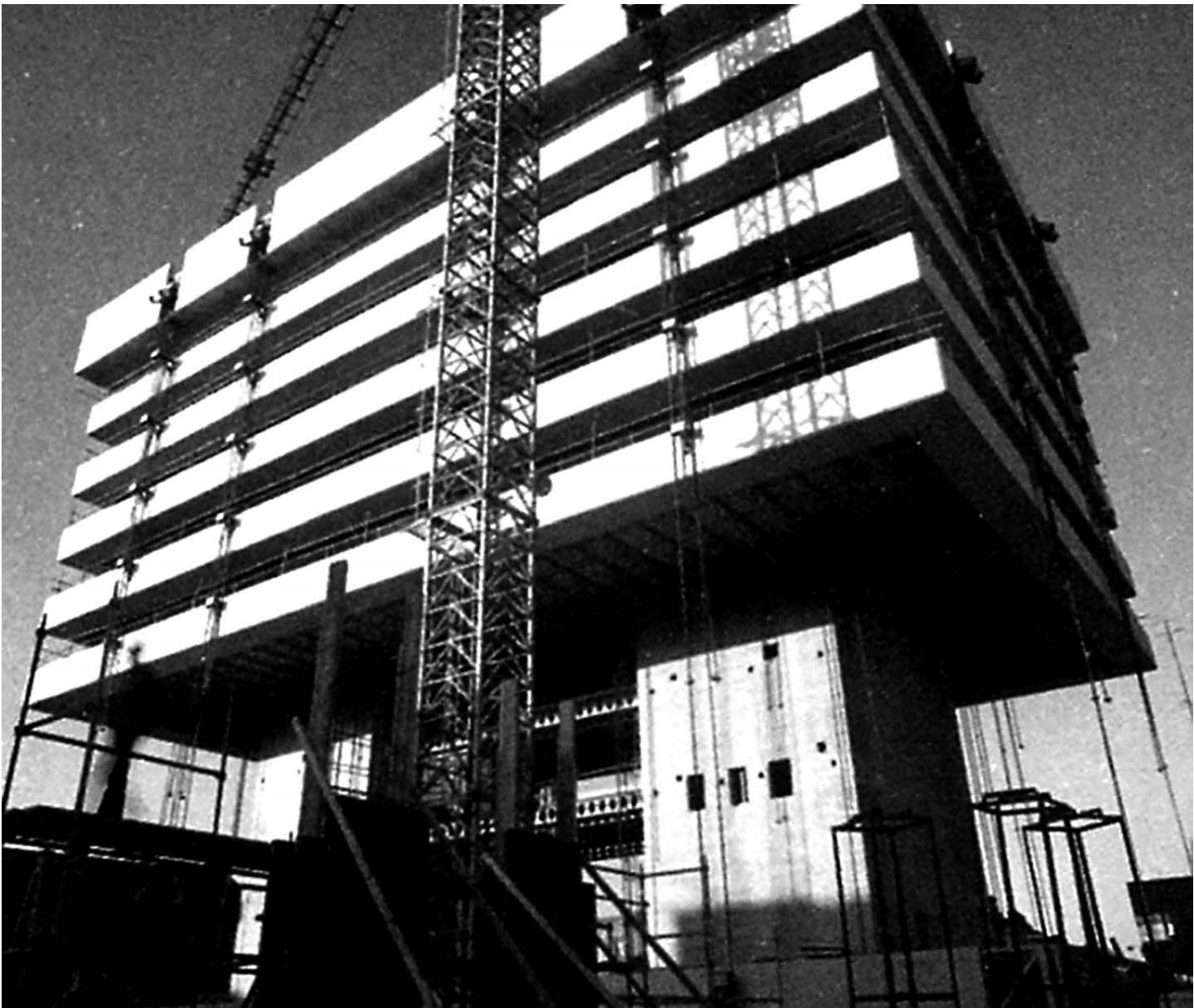
1974, ON THE BUILDING SITE, HOISTING UP THE FLOORS
