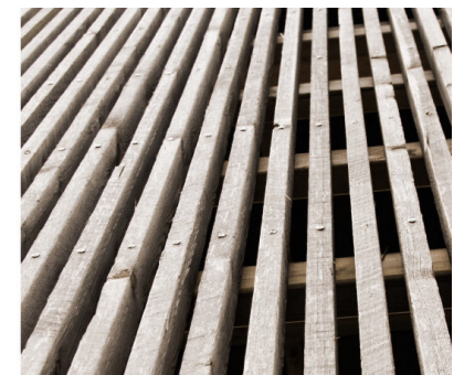
THICK PINE TRELLIS, FACADE ELEMENT AND IS ALSO USED AS RAILING SYSTEM IN SOME STAIRS AND TERRACES.
